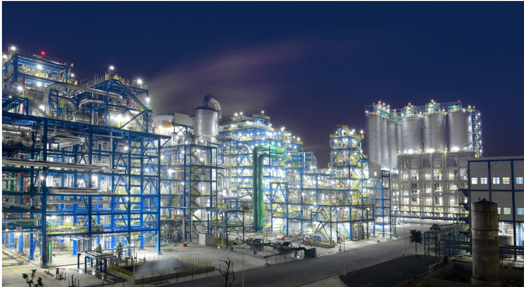
The night view of the second PTA line of China Prosperity (Jiangyin) Petrochemical Company Limited
